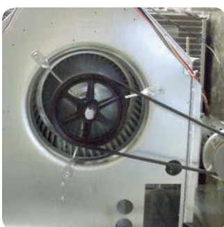
PowerMax DriveN Pulley on a Centrifugal Fan.
